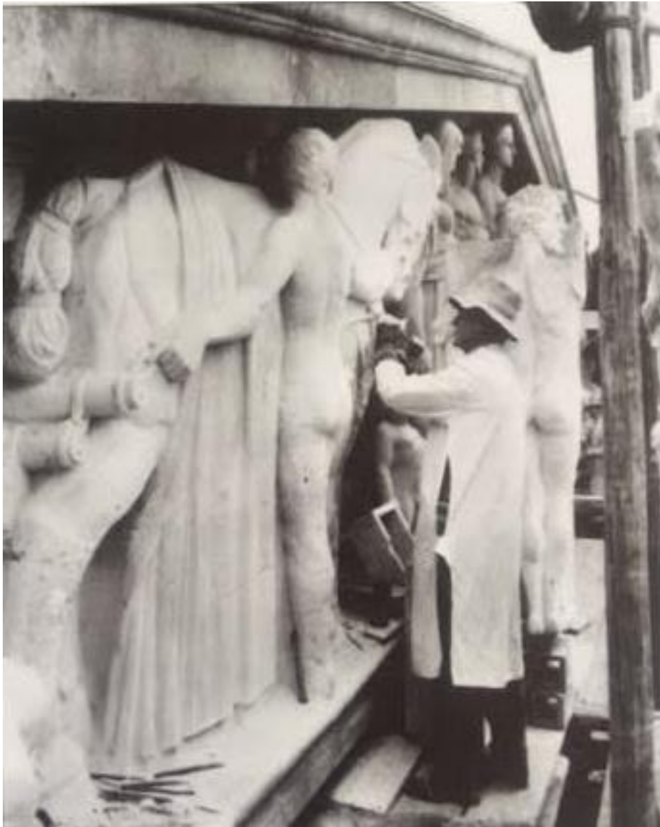
Working on the pediment of the Council House 1929.
