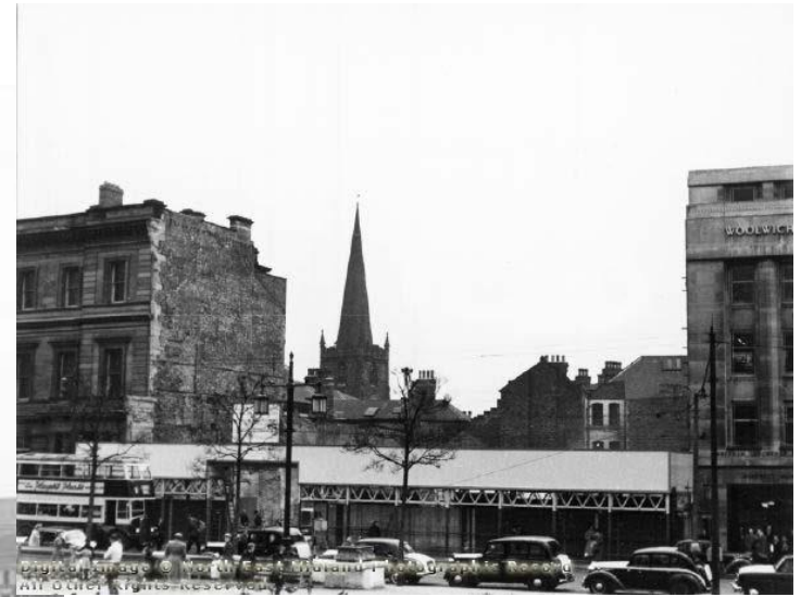
Foundations being built 1957.
