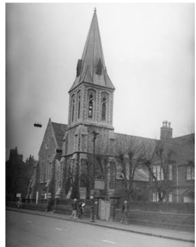
Figure 1: St Saviour's Church
