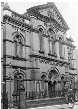
Figure 2: Castle Gate Congregational Chapel
