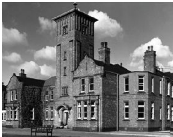
Figure 3: City Hospital Administration Block
